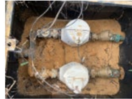
Meter with Dual Check Device
